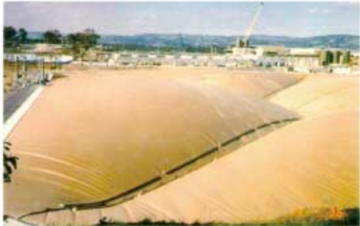
Burke Design Floating Cover: Potable water reservoir, Australia. Bottom Left: Inspecting reservoir under inflated cover. Bottom right: Access hatchway.
