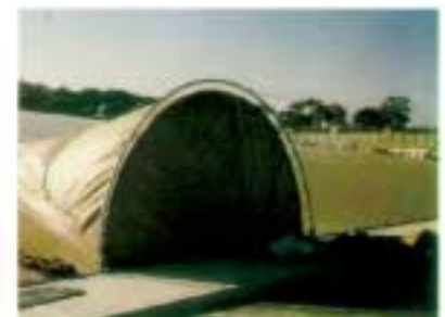
Burke Design Floating Cover: Potable water reservoir, Australia. Bottom Left: Inspecting reservoir under inflated cover. Bottom right: Access hatchway.
