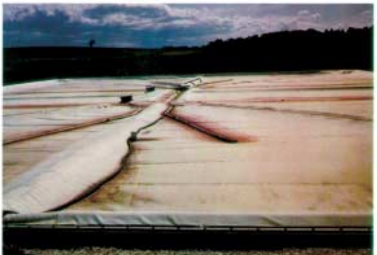
Cover: Methane gas collection system, Adelaide, South Australia.
