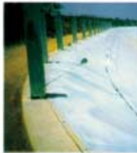
Tensioned cover, reservoir, Poway, California Left: Revoc Mechanical Tensioning System.
