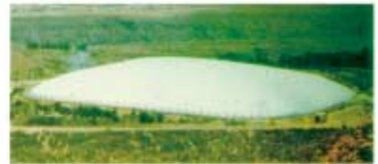
Tensioned cover, reservoir, Poway, California Left: Revoc Mechanical Tensioning System.
