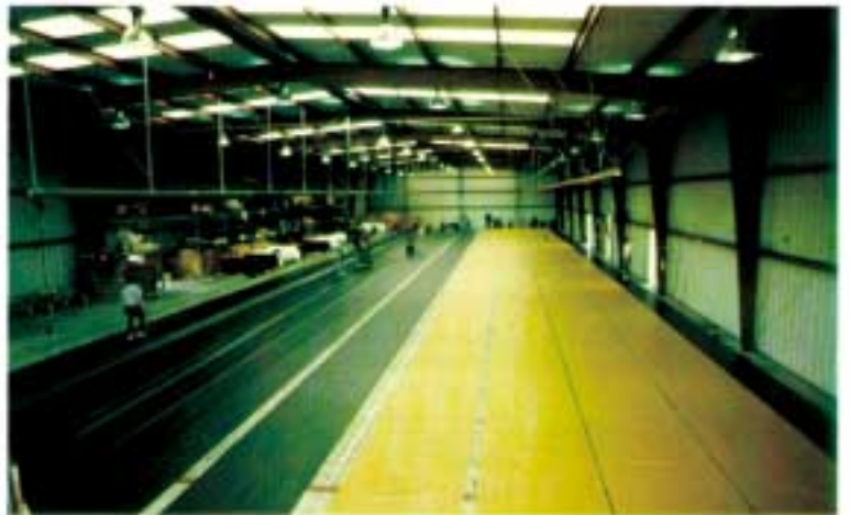
Burke custom fabrication plant, San Jose, California
