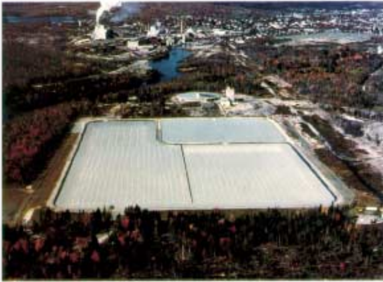
Liner: Pulp waste treatment lagoon, Great Northern Paper Co., Millinocket, Maine.
